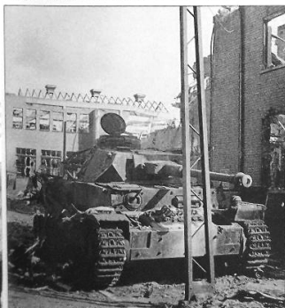
The two Pz.Kpfw.IV's that were photographed were already obsolete by September 1944, even though they had been modified. Both had been fitted with the new skirt attachment system but neither had zimmerit. The Pz.Kpfw.IV that came to its end under the pipe bridge had a new type tank commander's hatch. (IWM HU46265)
