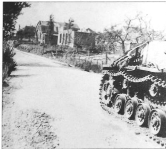
This Sturmgeschütz was successfully brought to a halt after at least eight direct hits. One completely removed the right differential gear housing. The hits also saw to it that the SP was entirely destroyed by fire. Despite the doubts about the number of tanks he put out of action, Baskeyfield made sure that, for a time, the Germans did not dare to advance any further. Fearful for the loss of more valuable armored vehicles, they preferred to keep their distance. (H.J. Wilink, Municipal Archives Renkum)
