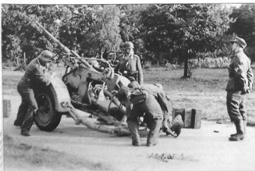
To prepare the gun for moving, the rear of the trailer had first to be hooked up to the mounting. Although this was only a small gun, this operation required four men. (BA 2K BK772/30)
