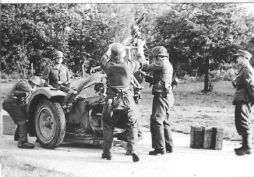
To prepare the gun for moving, the rear of the trailer had first to be hooked up to the mounting. Although this was only a small gun, this operation required four men. (BA 2K BK772/30)
