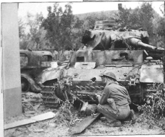
A little further back was this Panzerkampfwagen III Ausf. G. This was the second tank to be knocked out. This rare old type had received two direct hits in the front, one by the driver's vision slit and one on the front armor. (IWM B10376)
