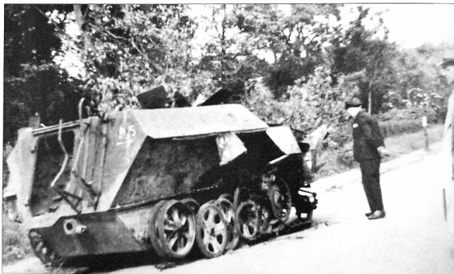
Here is the same SPW photographed from the other side in 1945. Although this armored half-track was a dangerous opponent for the parachutists, it could be stopped. Once in position with their anti-tank guns or PIAT anti-tank weapons it was possible for them to penetrate the relatively light armor plating. This Sd Kfz 250 was hit on the right-hand side just behind the track drive sprocket. It is not easy to see but the completely displaced roadwheels and destroyed storage box make this a fair certainty. (John A. Deweyert, Municipal Archives Renkum)
